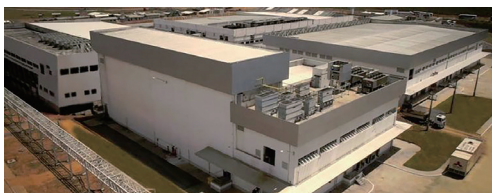
Figure 2 Hemobras plasma warehouse building.
